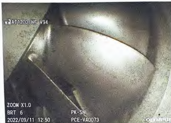
Photo of First Stage Compressor 3 rd Quadrant
