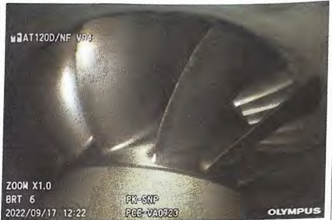
Photo of First Stage Compressor 4 th Quadrant
