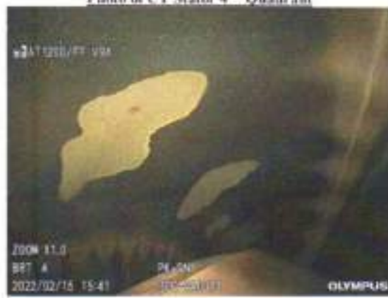
Photo of CT Stator 4 th Quadrant
