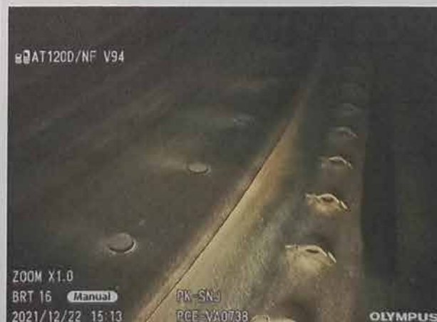
Photo of Combustion Chamber 4 th Quadrant
