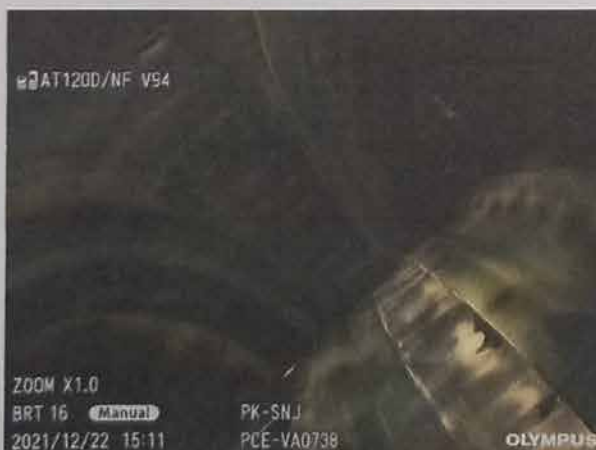
Photo of Combustion Chamber 3 rd Quadrant
