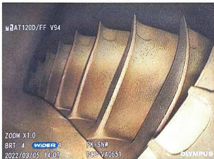
Photo of Leading Edge CT-Blades 1 st Quadrant
