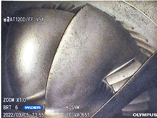
Photo of First Stage Compressor 3 rd Quadrant
