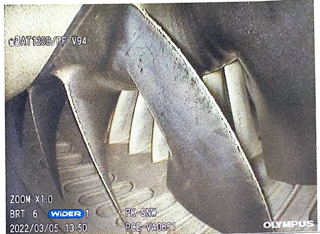
Photo of First Stage Compressor 4 th Quadrant
