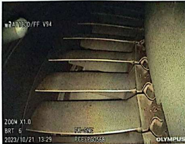
Photo of CT-Blades Trailing Edge 3 rd Q
