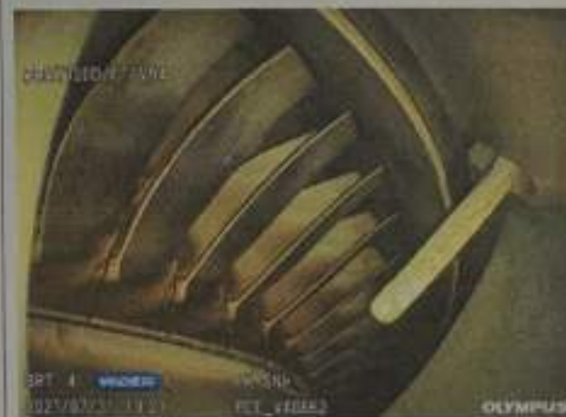
Photo of Trailing Edge CT-Blades 1 st Q
