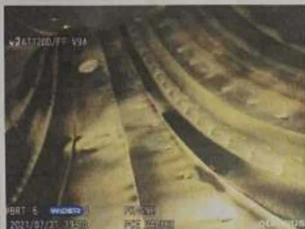
Photo of Combustion Chamber 1 st Quadrant
