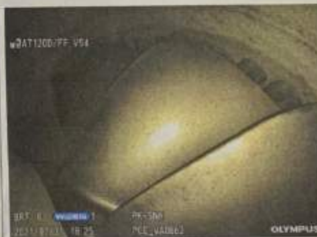
Photo of First Stage Compressor 2 nd Quadrant
