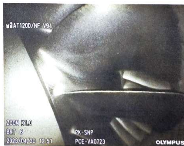
Photo of First Stage Compressor 2 nd Quadrant
