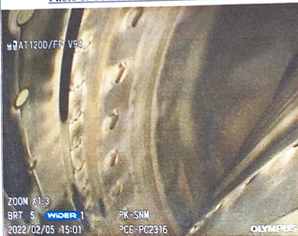
Photo of Combustion Chamber 1 st Quadrant
