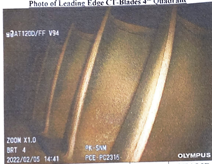
Photo of Leading Edge CT-Blades 4 th Quadrant
