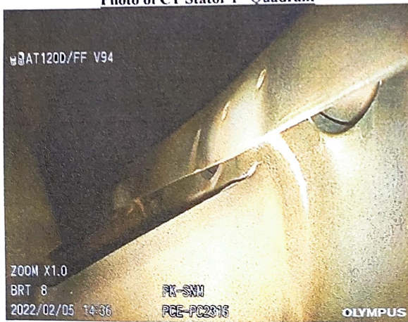
Photo of CT Stator 1 st Quadrant
