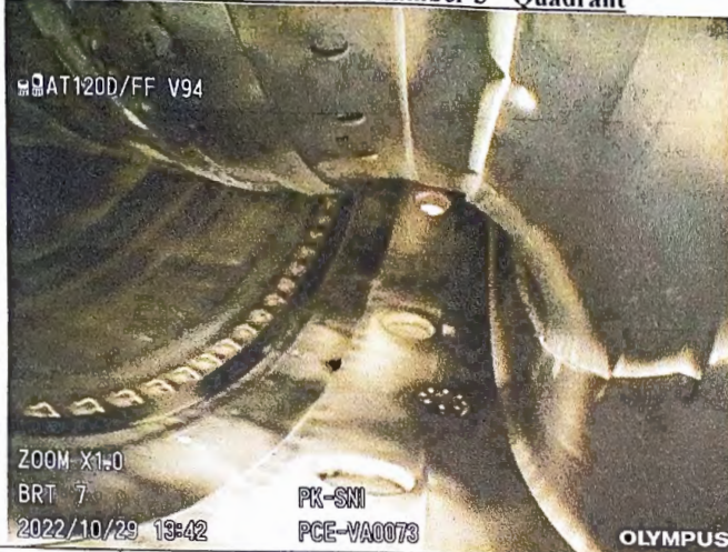
Photo of Combustion Chamber 3 rd Quadrant
