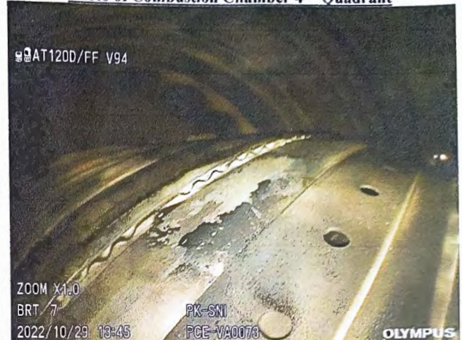
Photo of Combustion Chamber 4 th Quadrant
