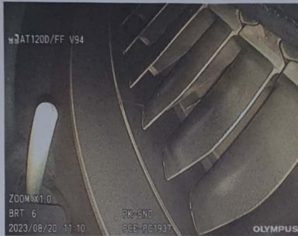
Photo of CT-Blades Trailing Edge 3 rd Q
