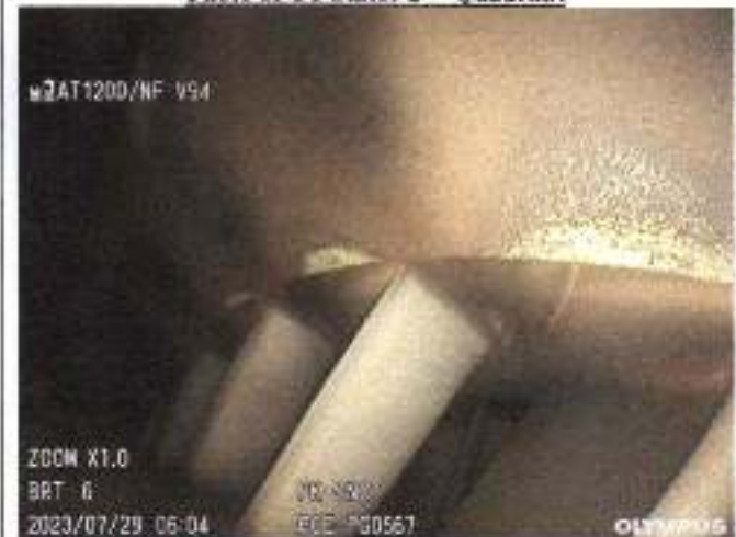
Photo of CT Stator 2 nd Quadrant
