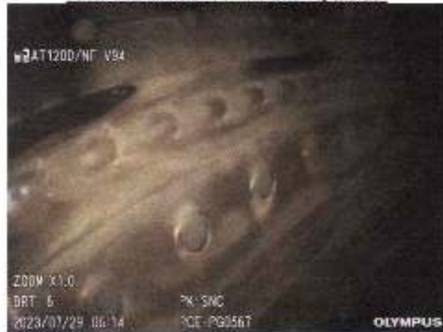
Photo of Combustion Chamber 3 rd Quadrant
