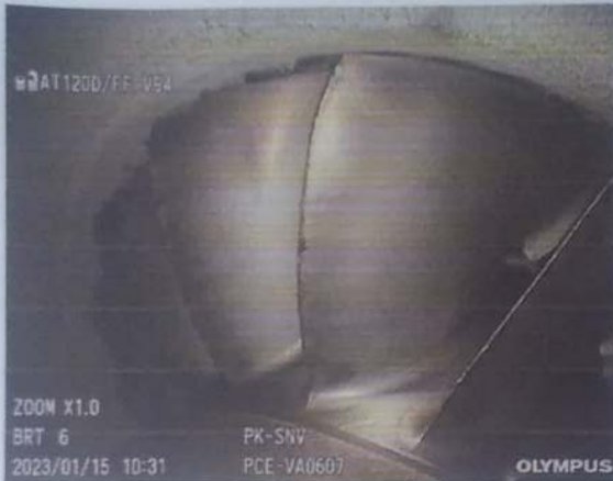
Photo of First Stage Compressor 3 rd Quadrant
