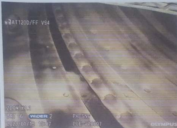
Photo of Combustion Chamber 3 rd Quadrant
