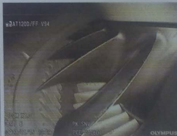
Photo of First Stage Compressor 2 nd Quadrant
