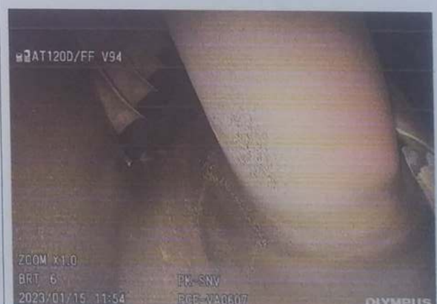
Photo of CT Stator 2 nd Quadrant
