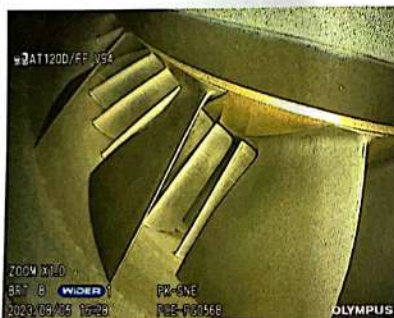
Photo of First Stage Compressor 1 st Quadrant
