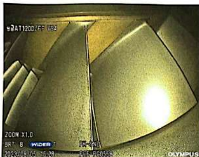
Photo of First Stage Compressor 3 rd Quadrant
