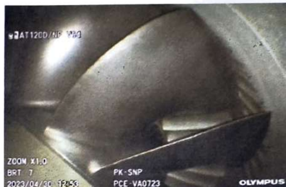
Photo of First Stage Compressor 4 th Quadrant
