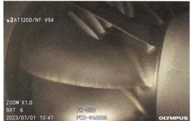
Photo of First Stage Compressor 4 th Quadrant
